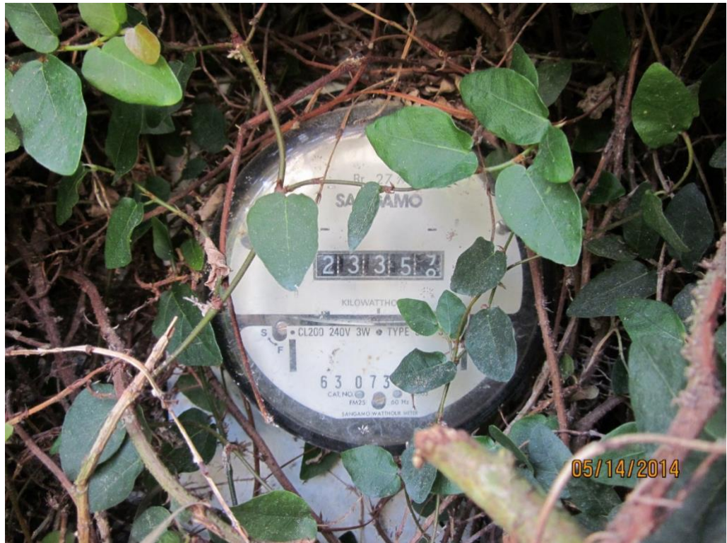
FIGURE 2.06C – REMOVE VINES 4' AROUND METERS AND ELECTRICAL DEVICES
